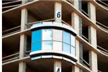
Unitised systems arrive at the site as fully prefabricated panels - glass and frame already assembled - ready to be hoisted and anchored
