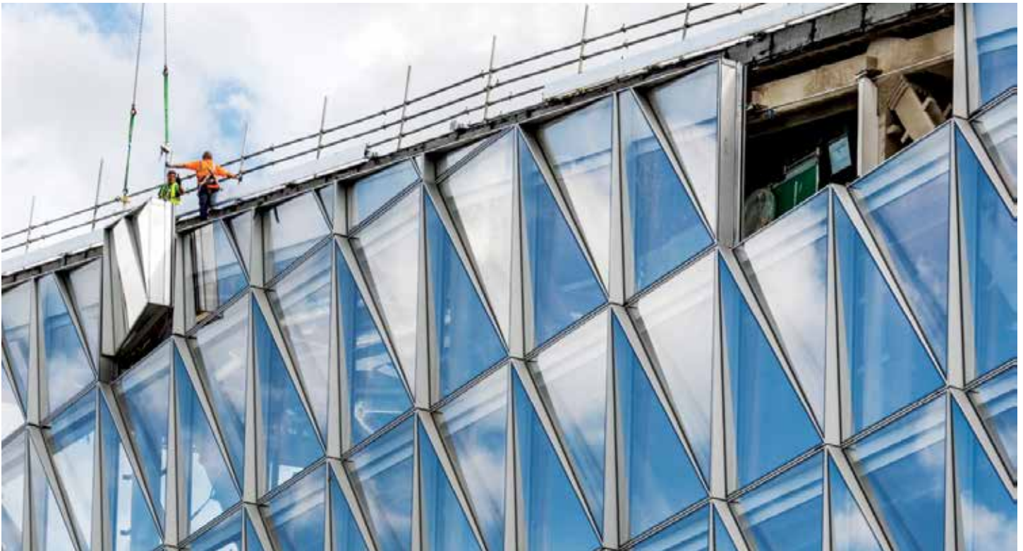
Unitised aluminium section semi for glass façade
